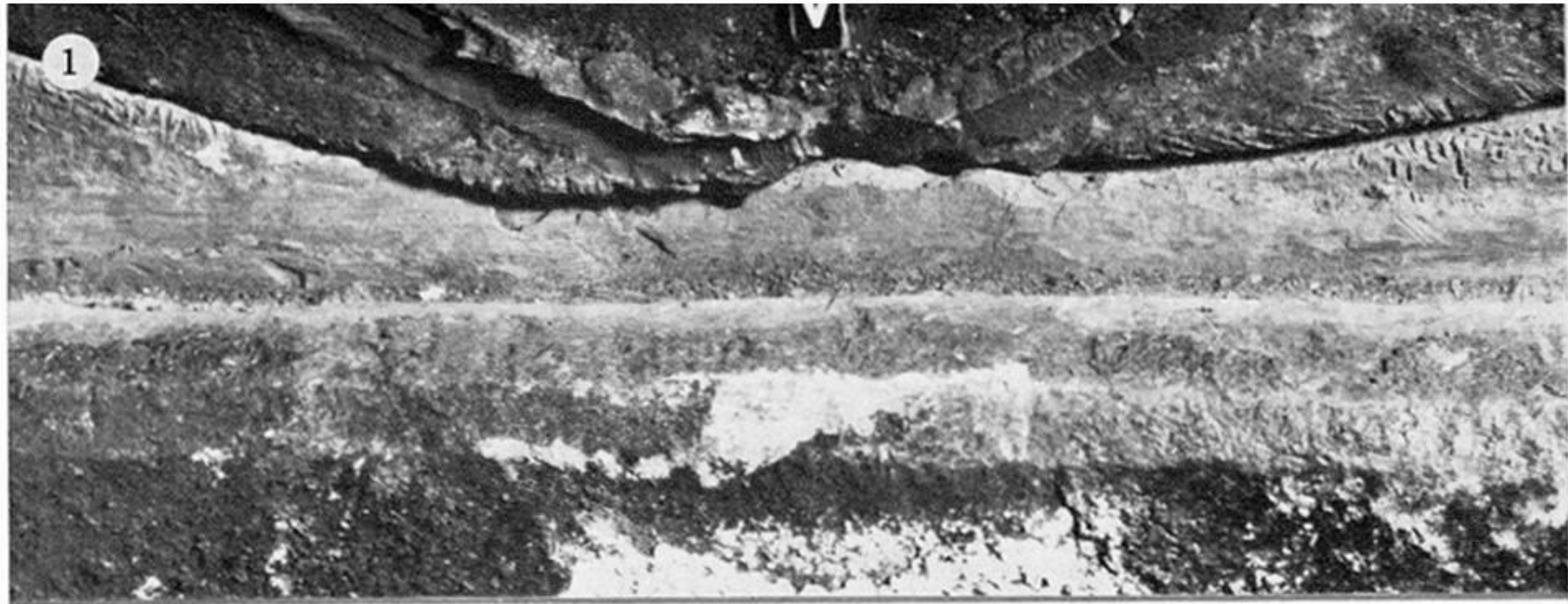
FIGURE 1. A major brittle fracture occurred in the deck of a cargo ship. This fracture started in a crevice between two close pitched fillet welded attachments to the deck plate. These were a thick plate type doubler and a tubular steel stanchion.
